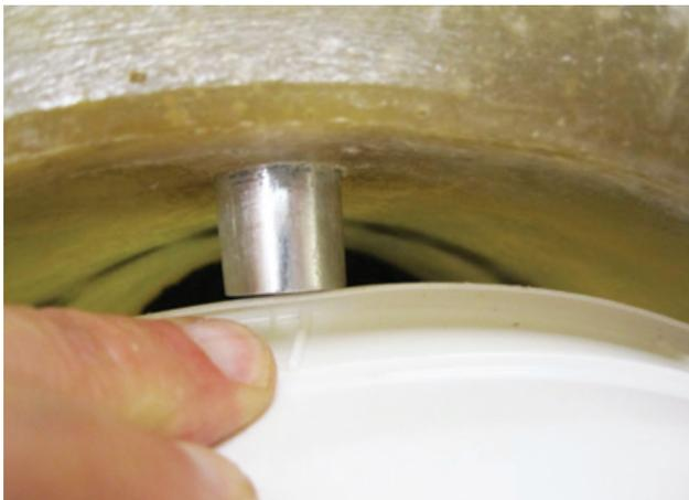
while avoiding the wire cage. If you sense any resistance from the cable and connectors, remove the pail- check that the wire cage and cables are positioned in the center of the pit. When properly positioned, the top of pail should be located below the level of the metal posts on the Dabico pit.
