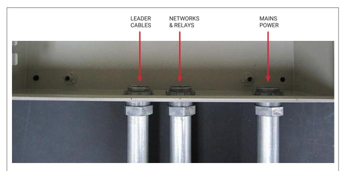
Figure 3. Example of completed conduit installation
