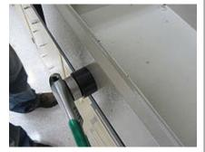
2. Install cable gland and conduit after holes are created. See figure below.
