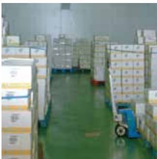
Freezer Frost Heave Prevention
